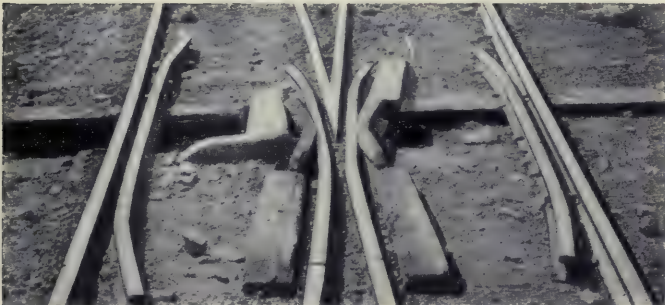
FIG. 17.—Tee rail shroud with spring.
